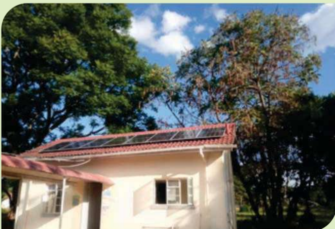
Rusape Hospital COVID 19 isolation centre
